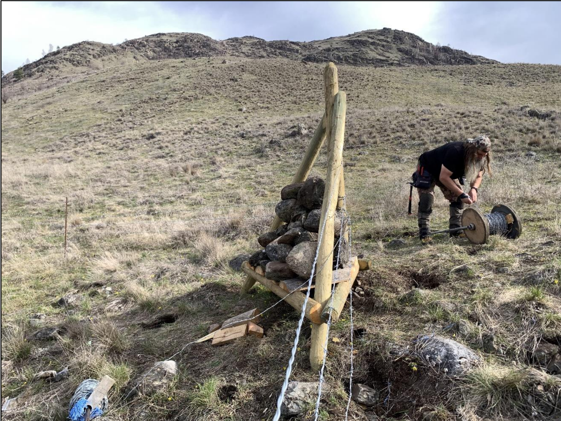
Figure 4: A rock jack corner brace on bedrock shows the amount of labour required to fence on difficult terrain typical of bighorn sheep habitats. Where in-line steel posts had to cross over bedrock, a 6-inch hole was first drilled into the rock (requiring a generator be moved to the site) and each post was then anchored into the rock with epoxy. These posts, each 1-inch in diameter, had to be cut-to-size to maintain proper wire spacing. This was all time-consuming and difficult work on steep and sometimes unstable ground. Thankfully, other than the relatively few but necessary wooden posts and rails, most of the new fence is fire-proof, substantively reducing the risk of infrastructure loss to future wildfires, an important climate-change adaptation.
