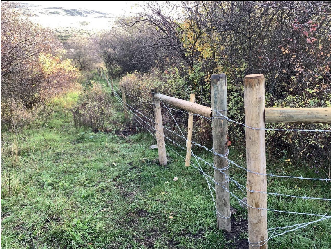
Figure 5: Livestock exclusion fence surrounding a waterhole and its riparian vegetation; the fencing has barbless top and bottom wires, with wires spaced to optimize wildlife crossings.
