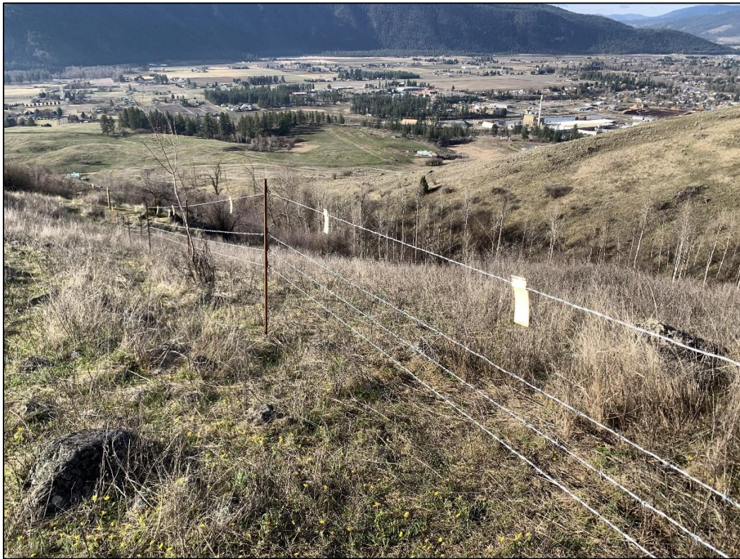
Figure 3: Installed wildlife-friendly property boundary fence; note the steel fire-proof posts, the low top and high bottom barbless wires, and vinyl flags added for wildlife awareness.
