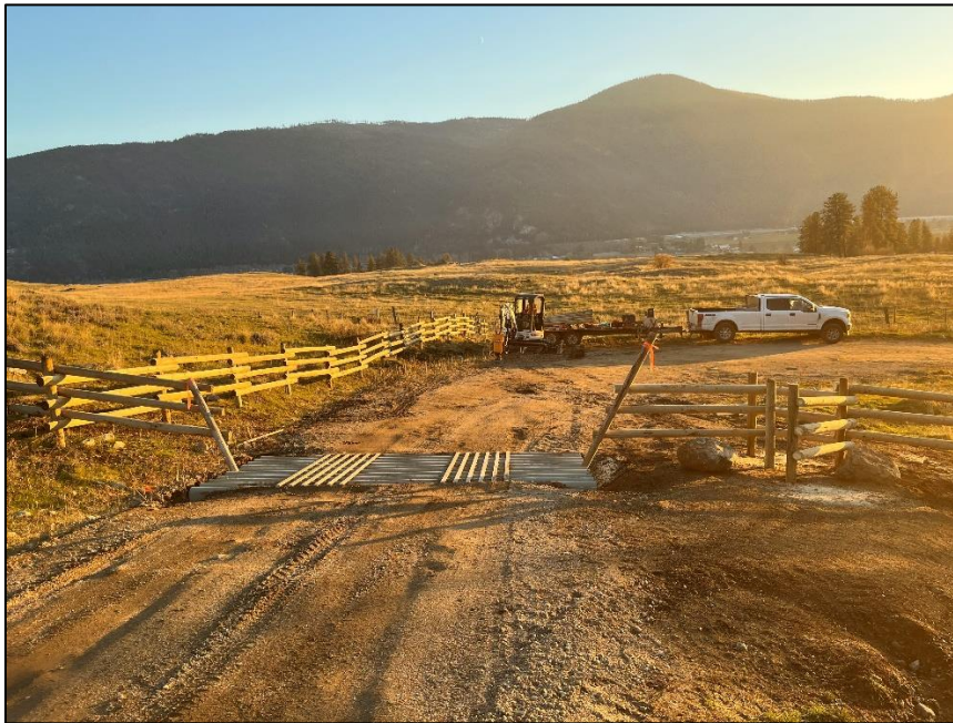
Figure 7: Cattleguard installed at the public road access to SILT's Grand Forks Grasslands conservation property. The rail wing fence makes the property boundary obvious. The top and bottom rails alternate to "wildlife-friendly" heights. A "crows-foot" provides pedestrian access without having to cross the cattleguard, and a locked farm gate in the far-left corner provides for removal of livestock that may find their way onto SILT's property in trespass. Property signage will be added in Spring 2024.
