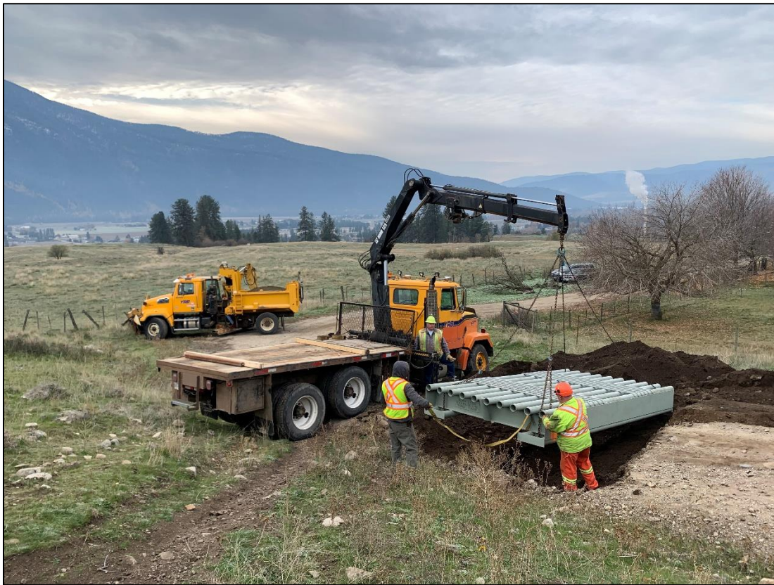
Figure 6: Cattleguard being installed on the public Morrissey Ck Road by YRB’s bridge crew.
